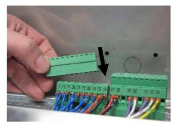
Replace the removable terminals wired to the male couplings mounted inside the cabinet on the DIN bar.
