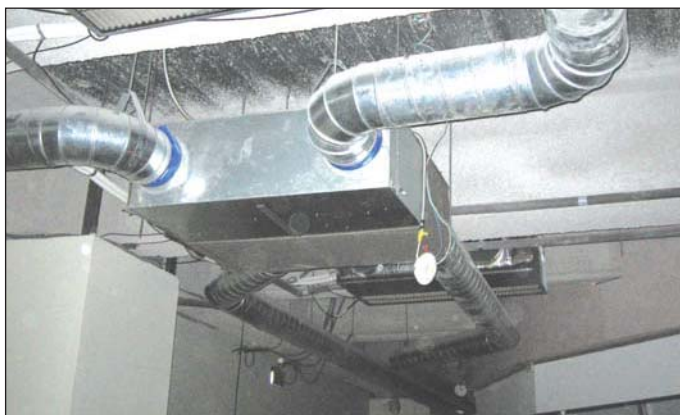
Lossnay installed in attic.
