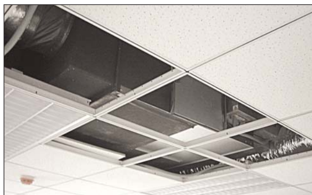
Lossnay installed in attic.
