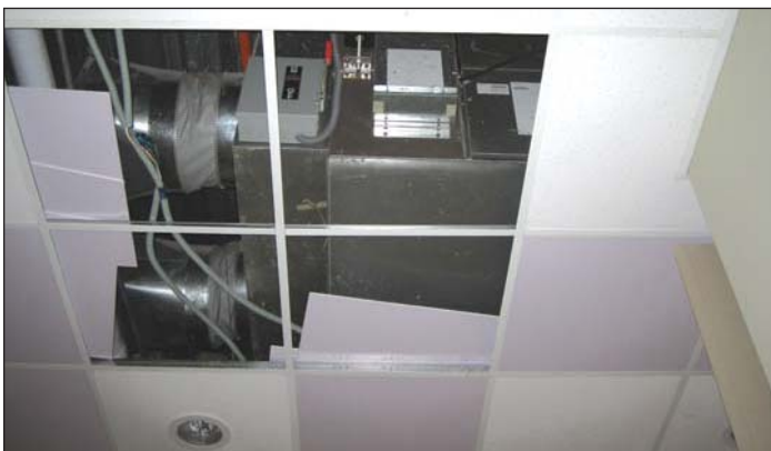
Lossnay installed in attic.
