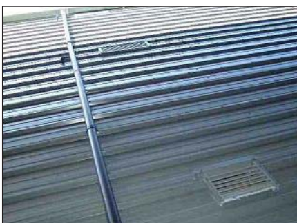
Weather cover is fixed the wall, it connected with duct.
