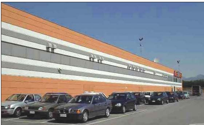
Weather covers are fixed the wall, it connected with ducts.
