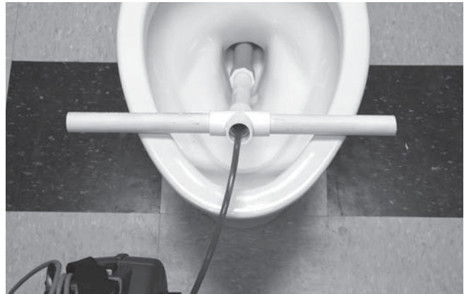
Figure 24 – Using A PVC Guide Tube
