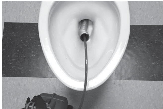
Figure 25 – Using The Flexible Guide Tube
