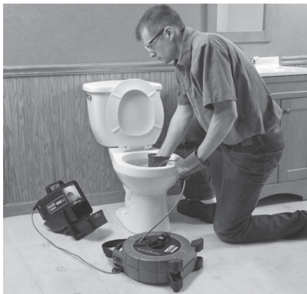
Figure 15 – Doing An Inspection
