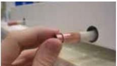
Mount a compression coupling and/or a valve to the pipe. Don't stress the nut too much, since this may crush the pipe.
