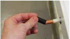
After removing the protection cover, make sure that the pipe is intact and undamaged, especially at the pipe end. Crocked or in other ways imperfect pipe ends will result in leaks. Deburr the pipe on the inside and the outside, using a deburring tool before installation
