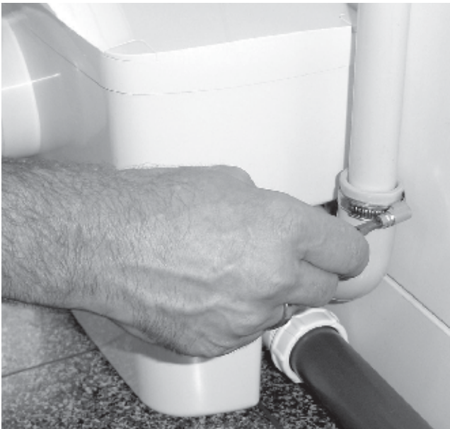
(Pic.4) To connect the pressure hose, please fasten the DN 25 pipe at the outlet bow, which is on the right at the tank of the Saniflux, with a clip. Install the pressure hose upwards (best way: first vertically, than horizontally) in a loop above the sewer level. This will avoid that waste water will flow back into the tank in case excess water (e.g. heavy rain) is in the sewer. Install the pressure pipe directly to the next soil stack. Please check again all connections and make sure that they are sealed. Now connect the unit with the power cable to the main supply and the unit is ready for operation.
