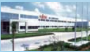
Fujitsu General (Shanghai) Co., Ltd.
