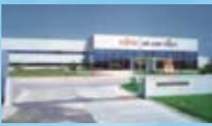
Fujitsu General (Thailand) Co., Ltd. Fujitsu General Engineering (Thailand) Co., Ltd.
