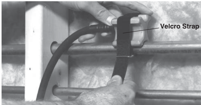
Figure 5 – Applying Freeze Head with Velcro Strap
