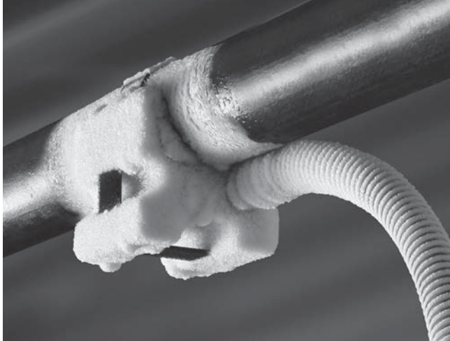
Figure 9 – Freeze Head Frozen to Pipe
