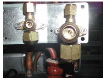
Figure 6.3 Liquid / gas service valve (Shown in figure is full open). (Operate with a hex-head wrench.)
