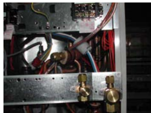
Figure 6.2 Service valve (Left: oil balancing tube, middle: Gas tube and the right: liquid tube)
