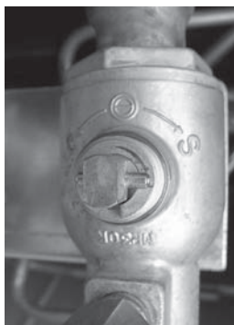
Fig. 6.10 Gas pipe Service valve (left figure) Liquid Service valve (right figure) <operate it with wrench> <operate it with hexagonal wrench> <the valve shown above is fully closed> <the valve shown above is closed>
