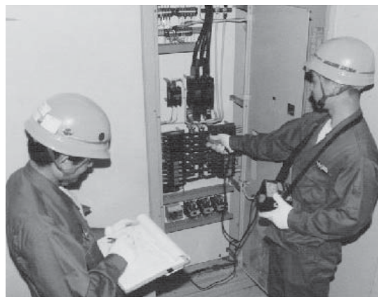
Fig. 6.12 Measuring insulation and power supply voltage
