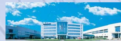
ПАНПАГЗ Panasonic Appliances Air Conditioning (Guangzhou) Co., Ltd.
