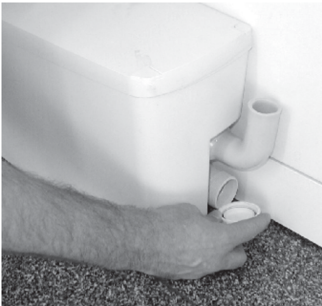
(Pic.1) Remove the cap, which is screwed at the inlet and take the black sealing ring and the white plastic ring out of the cap.
