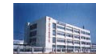
Hitachi Air Conditioning & Refrigerating, Китай
